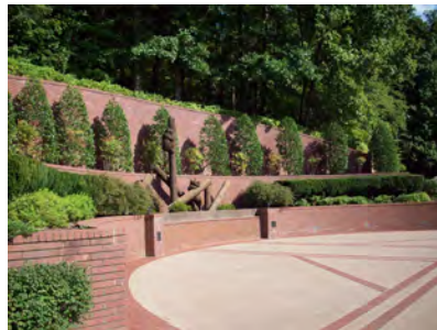
REAR RETAINING WALL/TURN-AROUND
