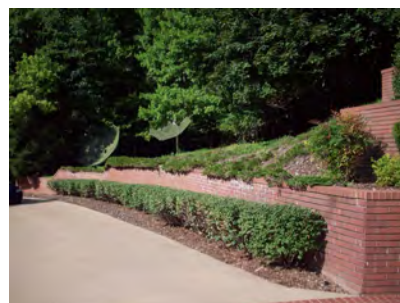
18. RETAINING WALL ALONG REAR OF DRIVE
