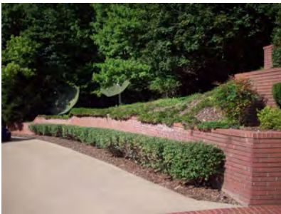
REAR RETAINING WALL
