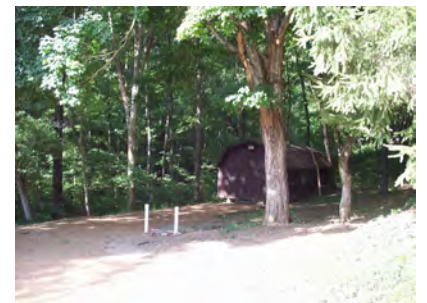
22. EXISTING STORAGE SHED
