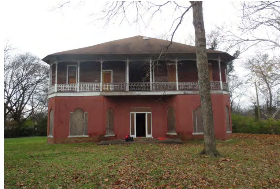
EAST FACADE OF THE MCGAVOCK HOUSE
