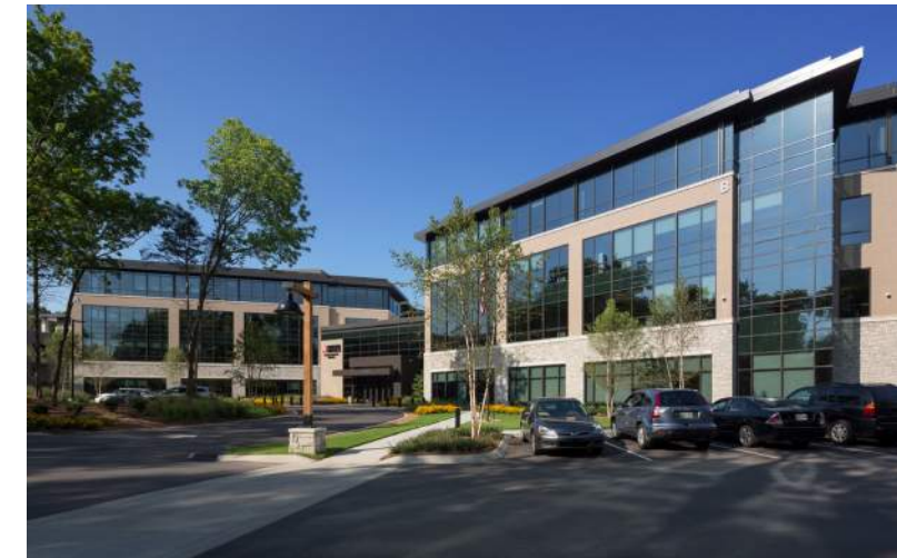
A Pedestrian Entrance Facade may be oriented toward and internal drive with parking beyond.
