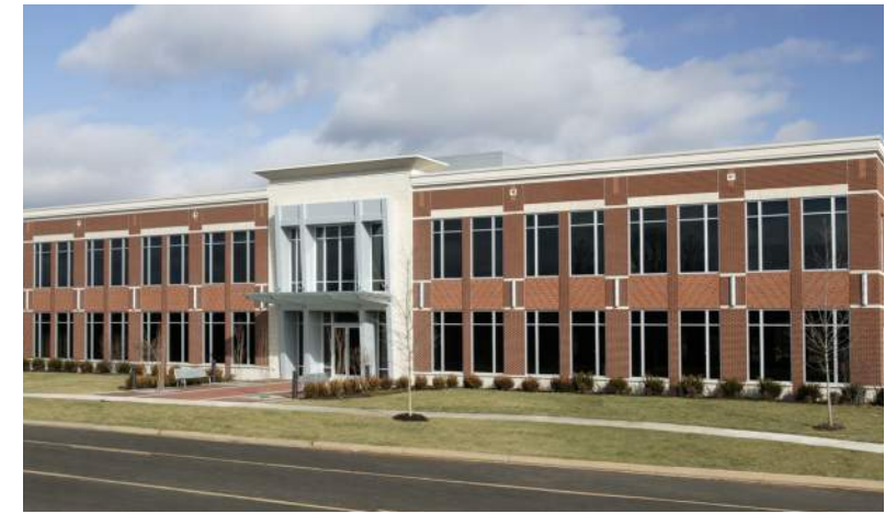
A Public Facade is oriented toward and Parkway or street. This facade has architectural interest and is the public face of the building to the community.
