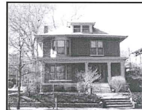
Within those portions of the Village featuring narrow buildings, a maximum building width requirement will be the key massing control.
