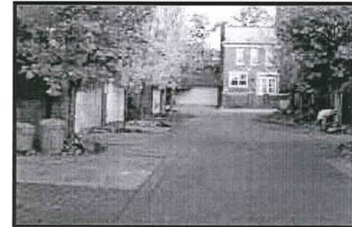
Alleys are necessary to accommodate rear parking. When well designed and maintained, they can be both functional and attractive.
