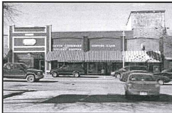
This central building has used pilasters and the shape of the parapet wall to divide a single facade into three vertically-oriented distinct bays which keep it in scale with neighboring buildings.
