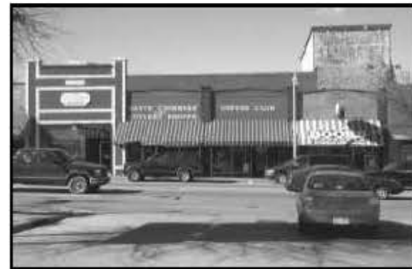
This central building has used pilasters and the shape of the parapet wall to divide a single facade into three vertically-oriented distinct bays which keep it in scale with neighboring buildings.
