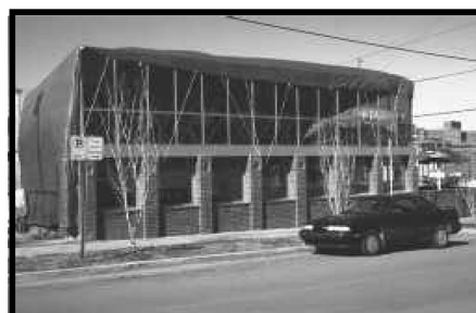
A wide variety of building types and designs characterize the commercial perimeter areas.
