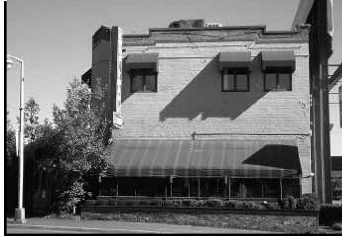
The Sportsman Grill is the only building identified as worthy of conservation in Sub-District 1C.
