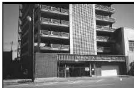
This garage detracts visually from its context and, without active ground-floor uses, can create dead spaces for the streetscape.
