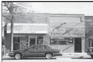
The building on the right has been altered by applying wooden panels to the base of the facade, thus obscuring the original brick.
