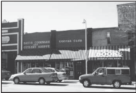
This building, located in Sub-District 1A, should serve as a model for future infill development.
