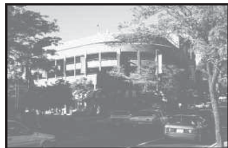
This parking structure has an architectural quality which looks more like a building, and the retail uses at the ground level help activate the streetscape.
