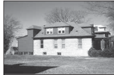
This low pitched, hipped roof with dormer windows is characteristic of American Foursquares and bungalows.
