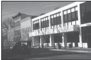
The color, materials and architectural detailing on the facade of this infill building are incompatible with the adjacent, older buildings.
