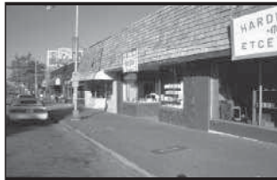
The false mansard roof in this image is too large for the building scale, inappropriate for the building's style, and obscures the building's facade.
