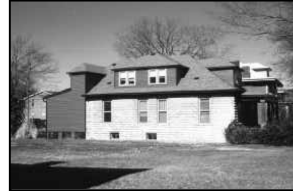
This low pitched, hipped roof with dormer windows is characteristic of American Foursquares and bungalows.
