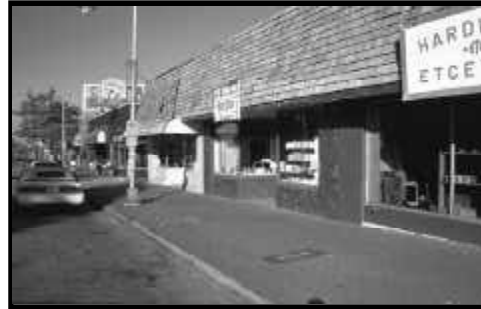
The false mansard roof in this image is too large for the building scale, inappropriate for the building's style, and obscures the building's facade.
