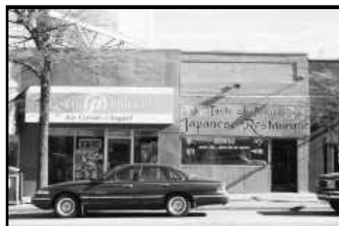
The building on the right has been altered by applying wooden panels to the base of the facade, thus obscuring the original brick.
