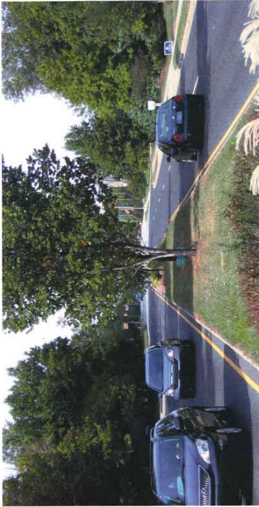
The Parkways in the development will have two travel lanes in both directions, a landscaped median to accommodate turn lanes, planting strips and sidewalks on both sides of the street. The design of the street will accommodate vehicular traffic and provide safe and attractive mobility for cyclists and pedestrians.
