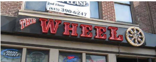
Example of raceway incorporated as sign background
