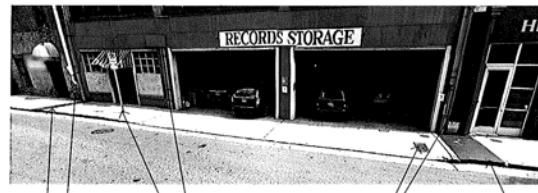
down spout electrical water metal drain cover metal drain cover sign down spout metal drain cover
